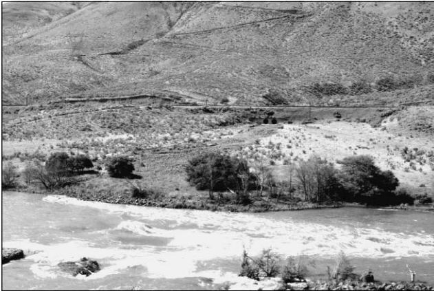
Figure 15. View north of the tributary fan at RM 7.8, where a July 1995 debris flow transported bouldery gravel into the Deschutes River channel, forming 'Washout Rapids.' Culverts under railroad have diameters of 4 m. June 2, 1998 photograph by J. E. O'Connor.
